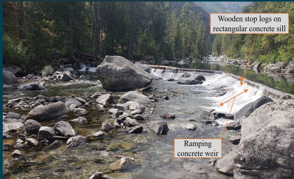
View of the gate house, conveyance channel, intake, sluiceway/fish ladder and diversion dam
